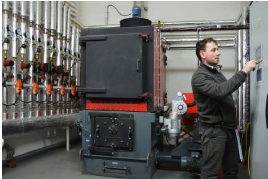
Automatic boiler room for wood biomass
